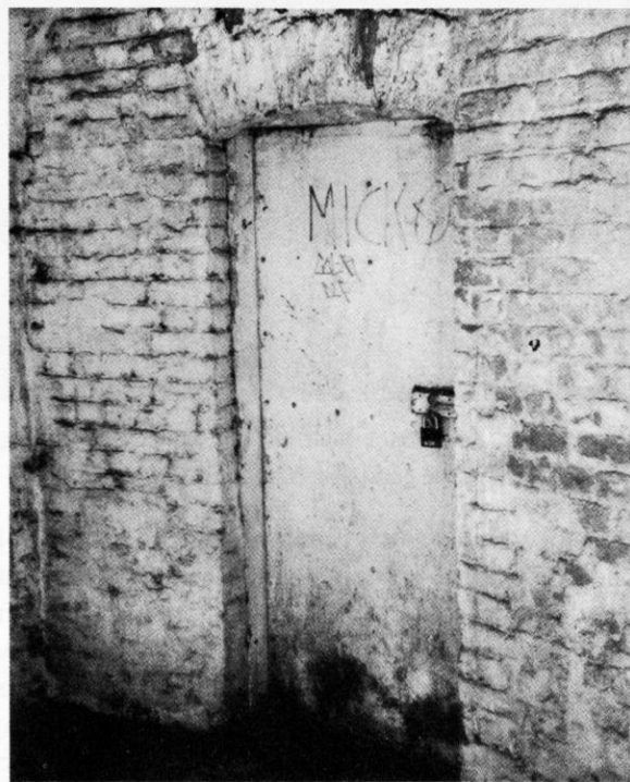
Iron door in east wall in June 2006 – Photo by Adam Sowan
